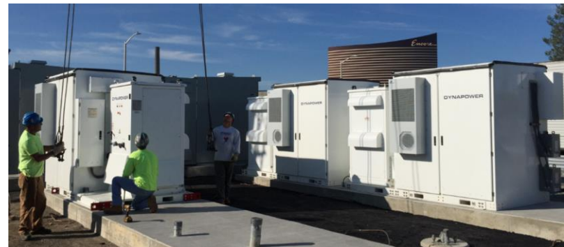
Largest BTM project at a commercial and Industrial building in the US (Boston)
