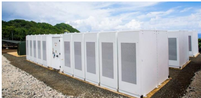
First island nation (TUA American Samoa) to run 100% on renewables
