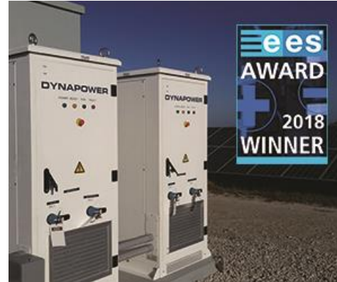
The US' first deployment of DC-coupled Solar Plus Storage (Florida)
